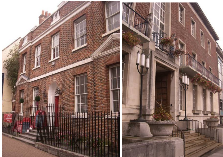
Figure 5.21 - Good building maintenance on High Street, Newport
