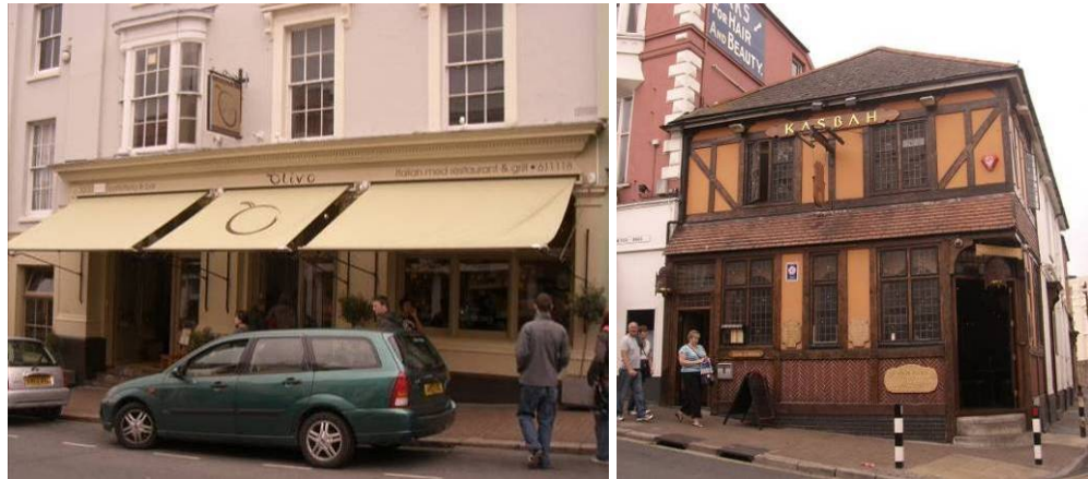
Figure 5.30 - Example of quality frontages on Union Street, Ryde.
