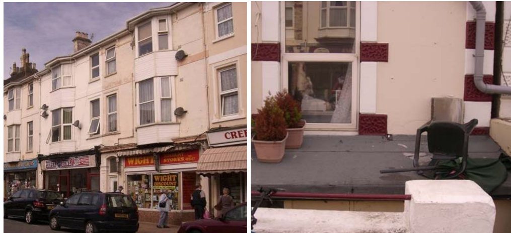
Figure 5.36 - Poor quality building frontages on High Street, Sandown
