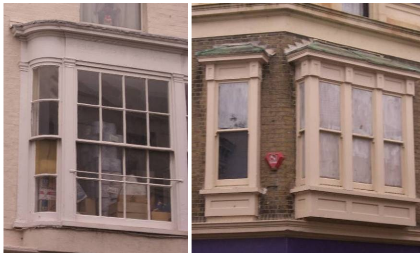
Figure 5.31- Under utilised upper floors on Union Street and High Street, Ryde
