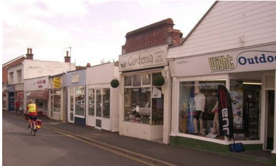
Figure 5.13 - 'Temporary' single storey retail units on Avenue Road
