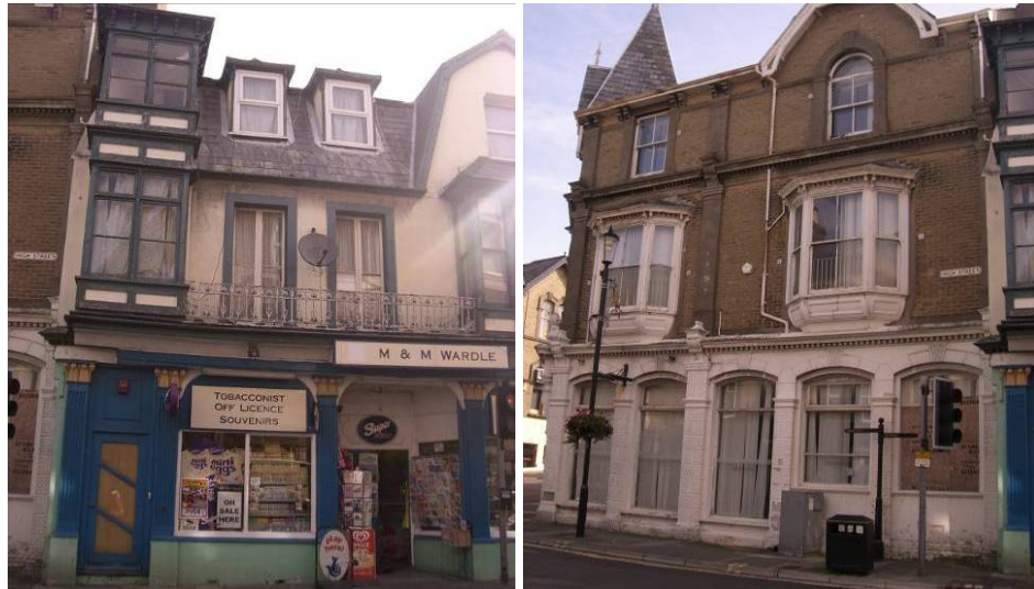
Figure 5.41 – Poor building and shop front maintenance on High Street, Shanklin
