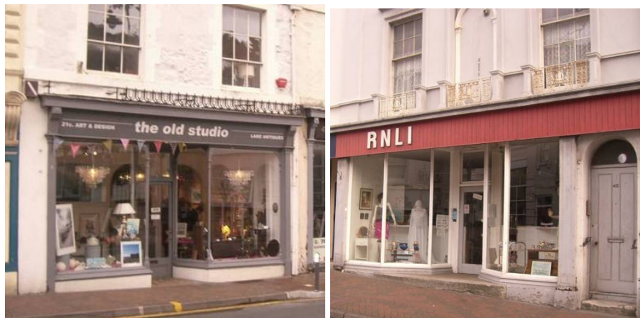
Figure 5.44 – Attractive shop fronts versus poor shop fronts on High Street, Ventnor
